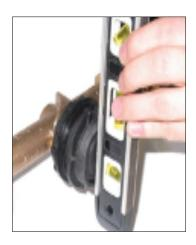
2. When installing the FAM Flow Tube with Plug, be sure to vertically level the Plug for future replacement with FAM Measuring Unit. Turn tap on to release any trapped air in line to the house/apartment. After air is released spot check for leaks around the installation
